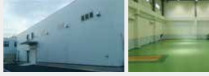
2nd Factory completed to improve working environment and double the production capacity 第二工場完成 生産能力2.5倍、作業環境を改善
